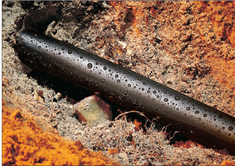
TREDUX HA47 - application below ground.
