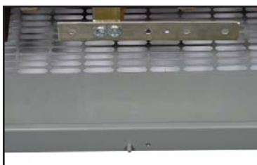
Bottom cable entry area where applicable
