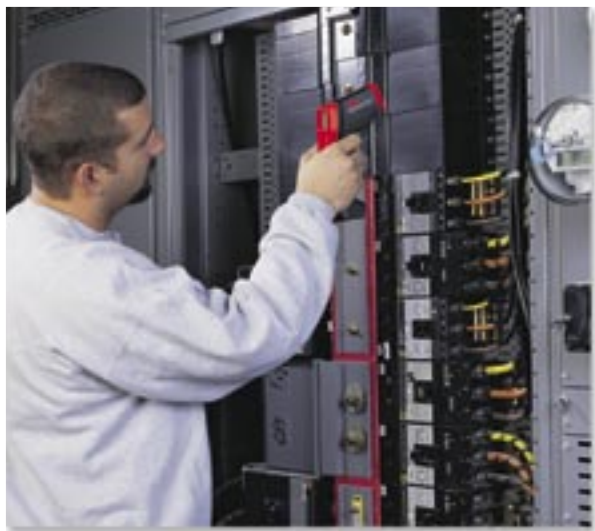
Check for hot spots in electrical panels and circuit breakers, generators and gearboxes.
