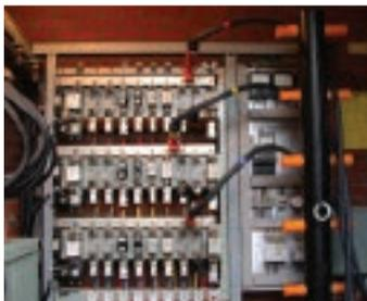
*Insulated G-Style clamps for direct connection to a live low voltage busbar.*
