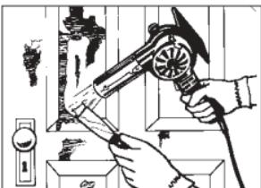
1) To strip paint, turn unit on and hold it about 1 inch from the surface being stripped. Proper distance and speed of stripping should be determined by experience. It is an advantage to hold the gun further from the surface and to move forward slowly. Slower speed is compensated by the wider softened areas. Heat will also penetrate deeper.
